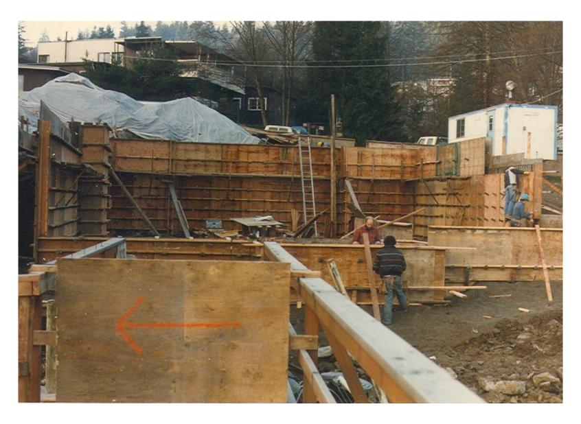
The forms for the basement concrete foundations - January 1985.
