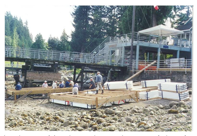
The three modules that make up the ramp dock under construction. A similar design was adopted for all docks constructed by the club. All lumber is 3" x 12" full dimensioned treated fir, with a 2" x 6" treated fir deck. The floatation consists of 30" x 60" X 20" deep plastic-wrapped polystyrene.
